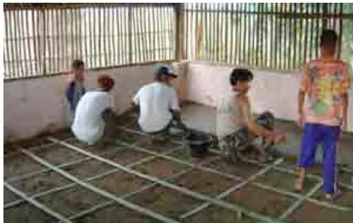
The staff and the older children of Childlife working together to lay the new floor.
