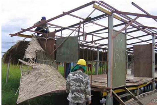
Volunteers from the Maesai District Office removing the old building.
