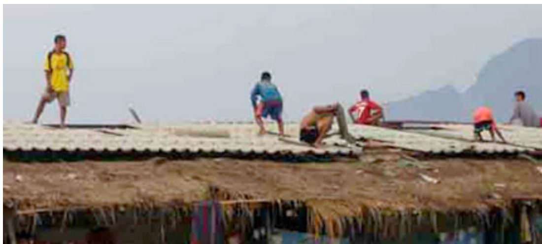
The children of Childlife attempting to repair the Shelter.
